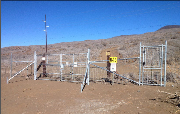
Example of a Vehicle gate with the appropriate braces in place.
