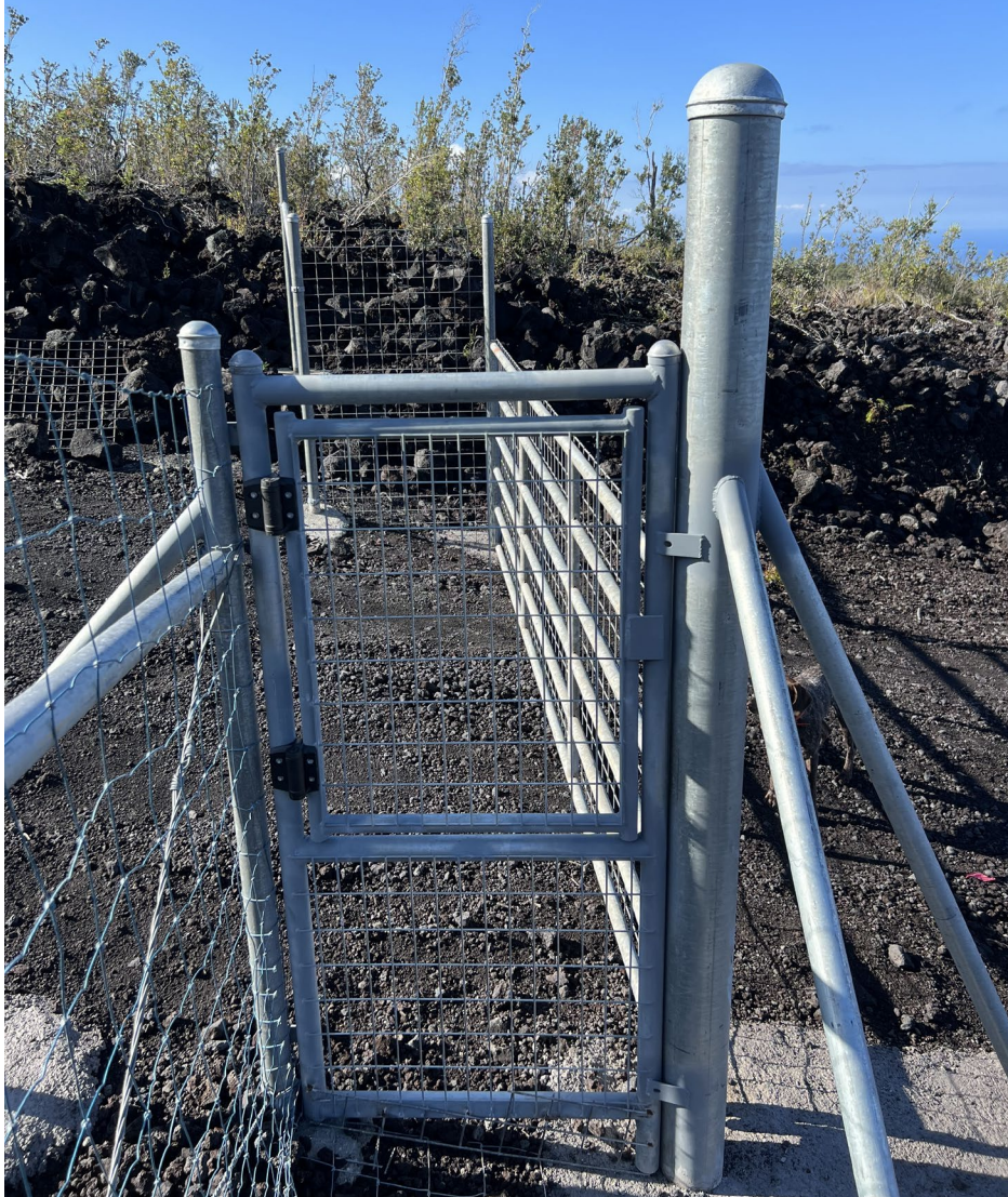
Pedestrian gate with appropriate braces in place
